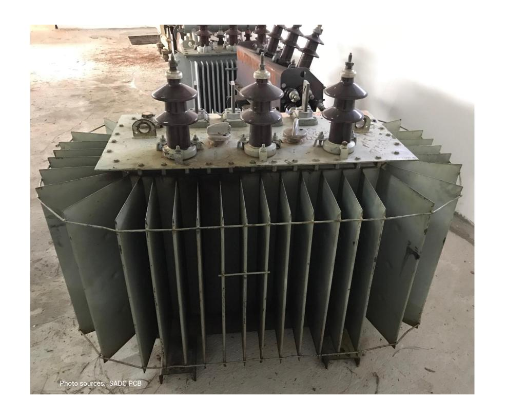
Many transformers built before the 1990s may contain PCB and have less energy efficient due to limited manufacturing techniques.
